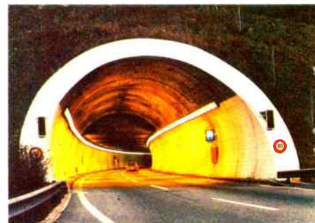
In Switzerland's Alps, thousands of GE lamps will soon help European motorists traverse the world's longest tunnel.
