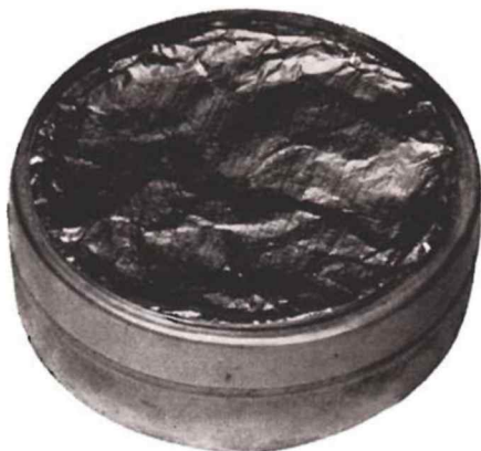
Fig. 1. View of Electrophone showing aluminum foil diaphragm
