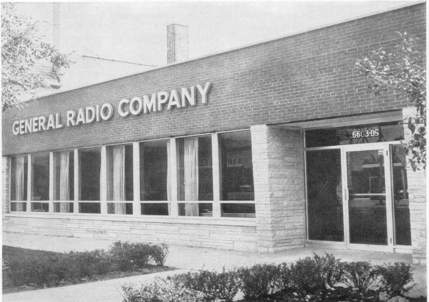
View of the new front door — 6605 West North Avenue, Oak Park, Illinois.
