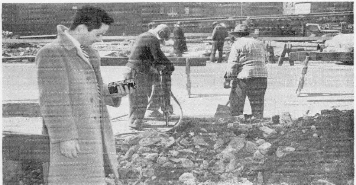
(Right) Figure 7. Sound-Survey Meter being used to measure noise level produced by pneumatic rock drills.
