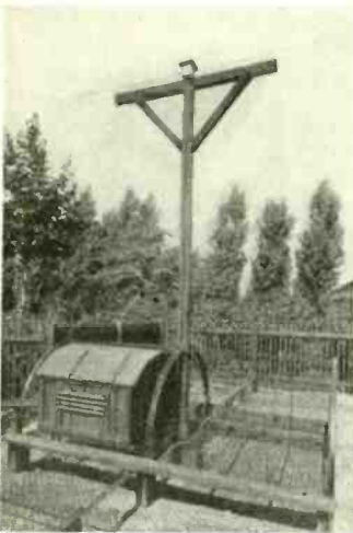
FIG. 9. THE COMPLETE SIGNAL TRANSMITTER SYSTEM. THE TRANSMITTER IS IN THE WOOD HUT UNDER THE REFLECTOR ARCH.
