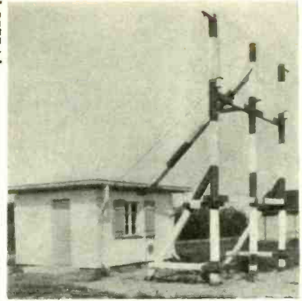
FIG. 6-B. THE RADIO BEACON GUIDE BEAM TRANSMITTER HUT WITH COMPLETE RADIATION SYSTEM. SEE FIG. 6-A.
