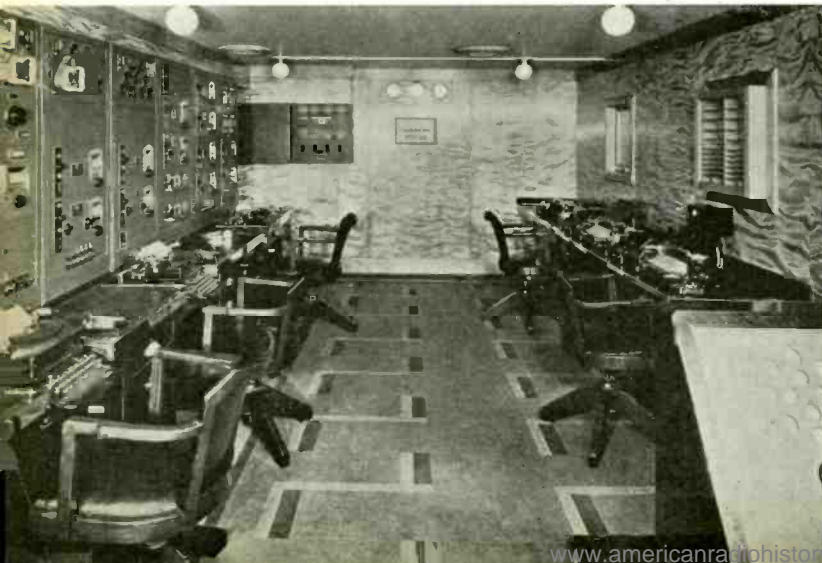
THE RADIO CONTROL ROOM.
