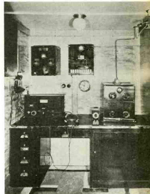
THE EMERGENCY EQUIPMENT COMPRISING TRANSMITTER, RECEIVER AND ACCUMULATOR BATTERY.
