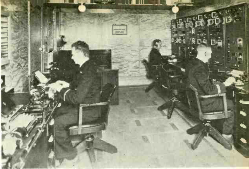
THE CONTROL ROOM SHOWING OPERATORS AT WORK.
