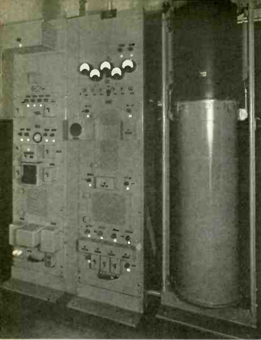
ABOVE: THREE-METER TRANSMITTER USED IN NEW ULTRA-SHORT-WAVE RADIO CIRCUIT CONNECTING NEW YORK AND PHILADELPHIA. RESONANT LINES ARE USED IN BOTH TRANSMITTERS AND RECEIVERS TO ELIMINATE NECESSITY FOR CRYSTAL CONTROL. RIGHT: FRONT VIEW OF ULTRA-SHORT-WAVE RECEIVER.
