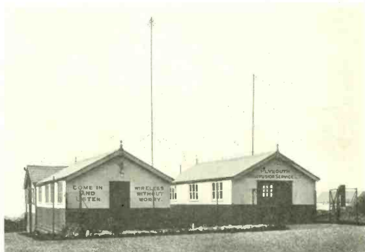
FIG. 1. A TYPICAL "REDIFFUSION" RECEIVING STATION.
