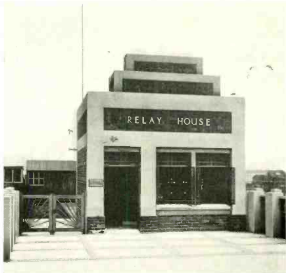
FIG. 4. EXTERIOR OF AN UNATTENDED SUB-STATION.
