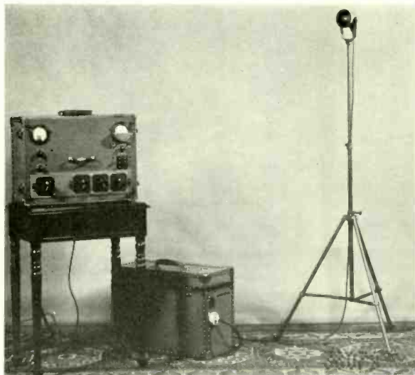
FIG. 1. A GENERAL VIEW OF THE HIGH-QUALITY REMOTE PICKUP EQUIPMENT DESCRIBED IN THIS ARTICLE. THIS EQUIPMENT CONSTITUTES A COMPLETE SPEECH-INPUT SYSTEM IN MINIATURE AND MAKES POSSIBLE QUALITY APPROACHING THAT OBTAINED WITH THE BEST STUDIO EQUIPMENT.
