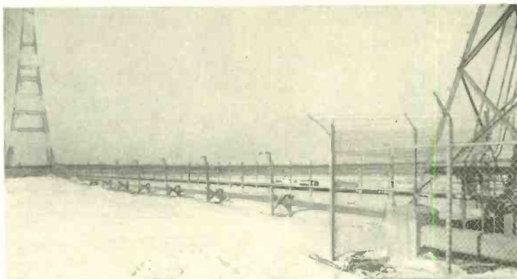
CATWALK, 790 FEET LONG, EXTENDING BETWEEN THE TWO ANTENNA TOWERS. THE CATWALK SUPPORTS ELECTRICAL CONDUITS AND THE CONCENTRIC TRANSMISSION LINE WHICH MAY BE SEEN JUST BELOW THE TOP RAIL. THE TRANSMISSION LINE IS ALSO SUPPORTED BY THE RIGHT ANGLE BRACKETS PROJECTING BEYOND THE RAIL.
