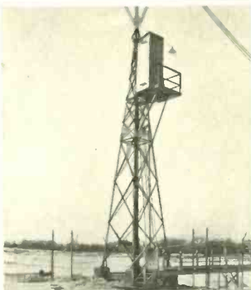
CLOSE-UP OF A SUPPORT LEG OF ONE OF THE TOWERS, SHOWING THE COUPLING HOUSE ABOUT 30 FEET UP WHICH CONTAINS THE TUNING EQUIPMENT FED FROM THE CONCENTRIC TRANSMISSION LINE THAT RISES TO IT FROM THE CATWALK.
