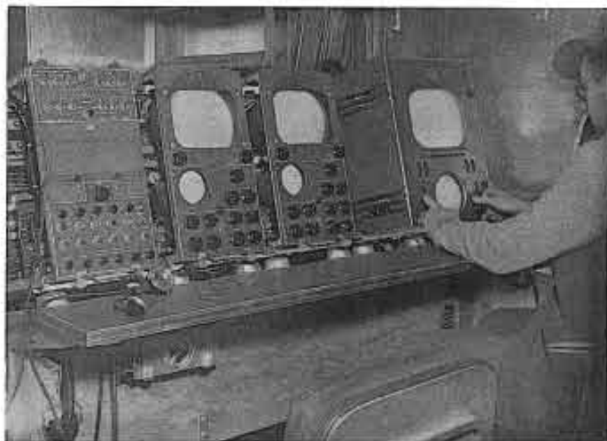
Figure 6 The video control desk. From left to right are the switching unit, two camera controls and space for a third, and a master monitor.
