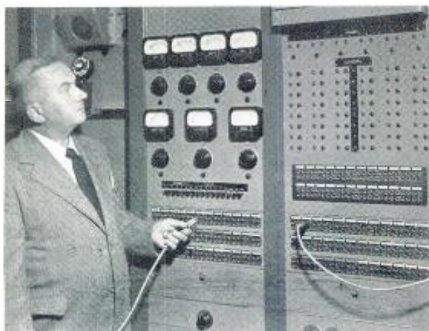
Charles Vassall checking a meter circuit in the master control board of the audio system at the WBZ Radio and Television Center. The volume indicator panel (left) gives a visible and audible check for entire standard band and FM studio setup, while the right bay provides for switching of eight studios and six channels.
