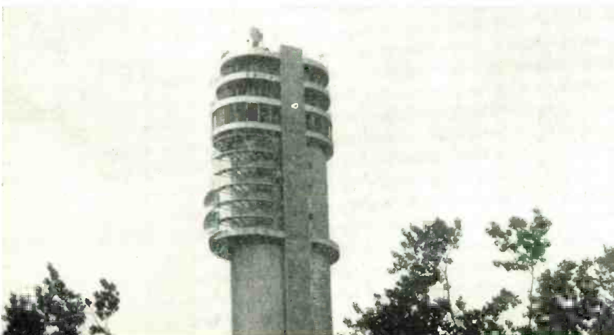
Below: View of the 300' microwave tower recently completed for the Federal Telecommunication Laboratories at Nutley, N. J. The tower houses experimental antennas and equipment for research and development work in television, aviation communications, multiplexing, microwave antennas, point-to-point communications, etc. Right: Three-bay RCA super turnstile tv antenna being mounted atop an RCA pylun 1-m antenna for WBZ-TV near Harvard Stadium, Mass. Tower is 656' high and designed to service an area of 40 miles radius of Boston.
