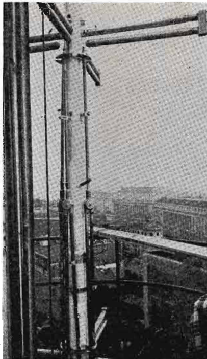
Above: Phasing, matching and feed lines required to produce a circular radiation field pattern. Rings into which the end seals fit are required to maintain a balance between the two transmission lines. Below: Closeup of overall antenna supporting structure. Front of the system is driven, while back acts as a parasitic reflector.
