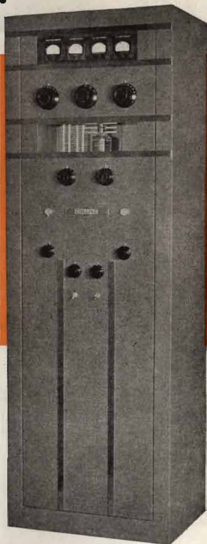
Collins 30K Transmitter
