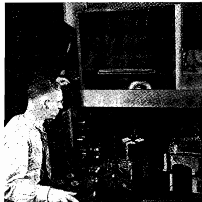
Karl Wendt with the trinoscope projection assembly of the recently-developed RCA electronic color television receiving system. The assembly consists of three 3" kinescopes to receive red, blue and green images.
