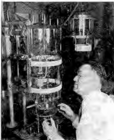
(Courtesy North American Philips Co., Inc.) Sealing anode and grid caps to bulb of an 833A with a h-f coil. Metal is heated by means of induction. Bell jar is filled with nitrogen to reduce oxidation.
