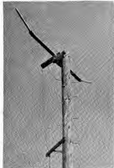
U-h-f doublet receiving antenna picking up signals from four Chicago f-m stations for observation.
