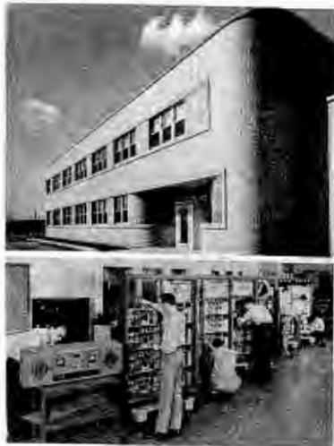
Top, the streamlined Motorola Engineering Building. Below, a research production line in this new building.
