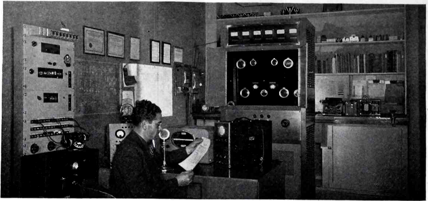
Central station KFCD in Los Angeles.
