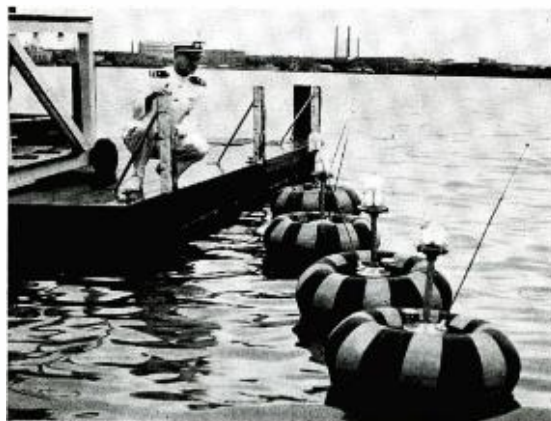
• • • Showing several of the radio - controlled sea drome lights. Note antenna and lights. • • •
