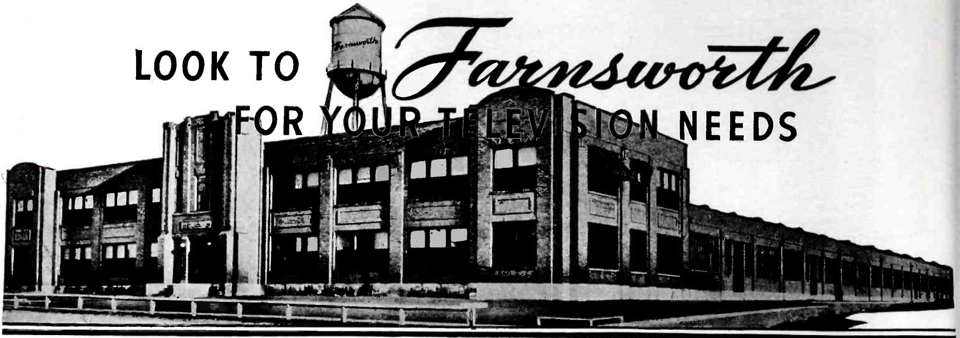
Farnsworth's Fort Wayne plant housing administration offices, research laboratories and special products manufacturing division.
