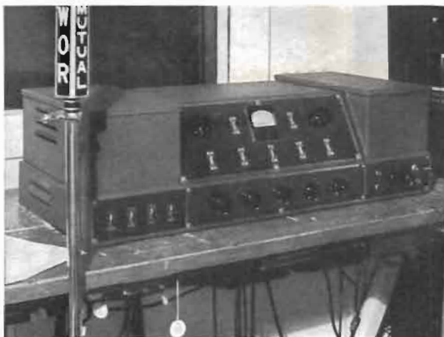
FIG. 8. The Type 23A speech-input console set up in a control booth of the Mutual Broadcasting System.
