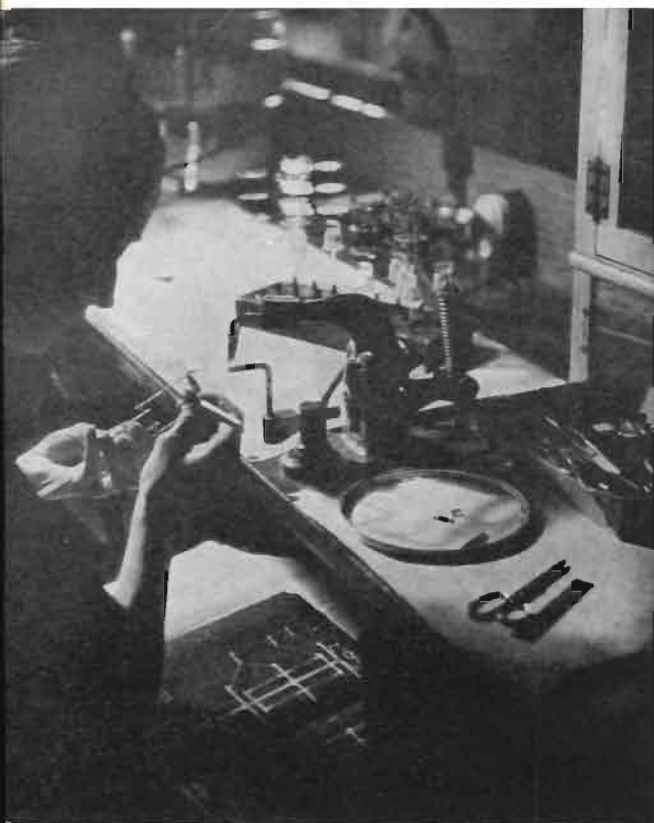
Deft fingers put the delicate filament in its suspending frame as an early operation in assembling the elements of a tube.
