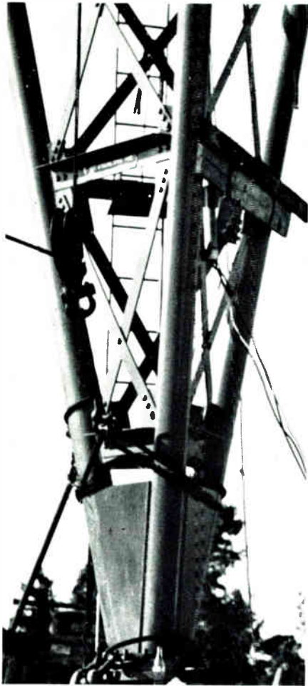
Typical anchorage for pivoted base type of guyed tower. Connected at a single point, the tower will remain upright and plumb even if the foundation shifts unevenly.
