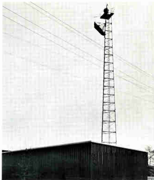
Self-supporting 135-foot microwave tower at Station WAVE-TV showing two receiving dishes on platform—one fixed and one rotatable. The reflector handles a 7000 MHz STL microwave and also a 2000 MHz STL, both with roof-mounted antennas.
