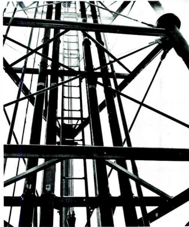
By placing a service ladder within the tower, the lattice braces form a safety cage for the servicemen.
