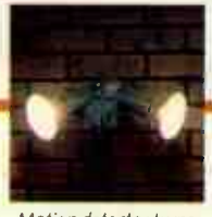
Motion detector turns on exterior and interior lights.
