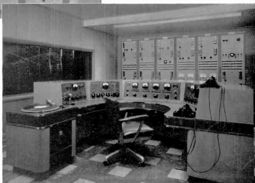
Master control desk, transcription turntable, and associated audio racks as installed at WISH, Indianapolis, Ind.
