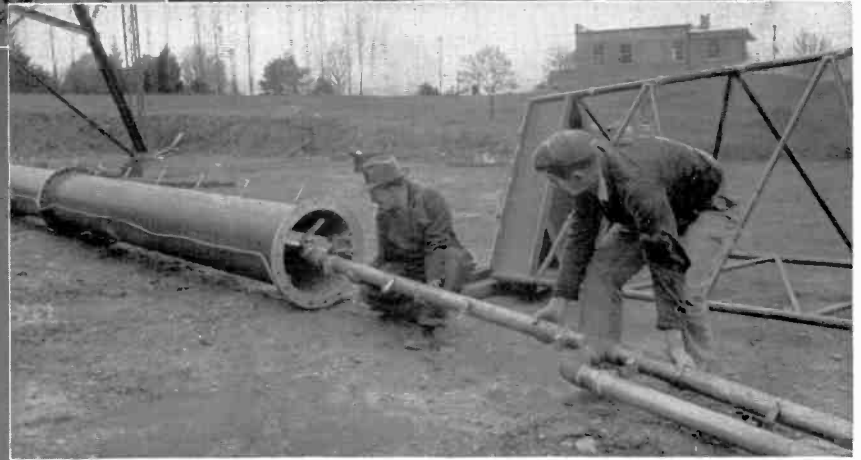
Inserting the transmission line harness into the two-section Pylon at WSBM-FM, York, Pa.
