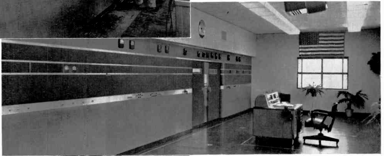
Fifty kilowatt transmitter, Type BTA-50F, with control console and extension cabinets containing phasing equipment, at KMPC, Hollywood, Cal.
