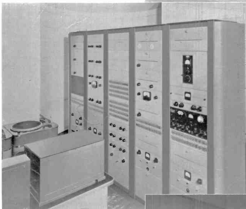
A partial view of the master control installation at WCAO, Baltimore, Md., showing the rack-mounted audio equipment. This is companion equipment to that shown on the opposite page top view.
