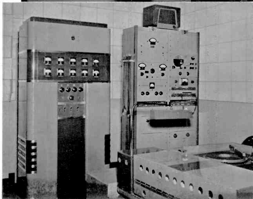
Control room at WMRN, Marion, Ohio, showing 250 watt transmitter, turntables, control console, and associated audio and test equipment.
