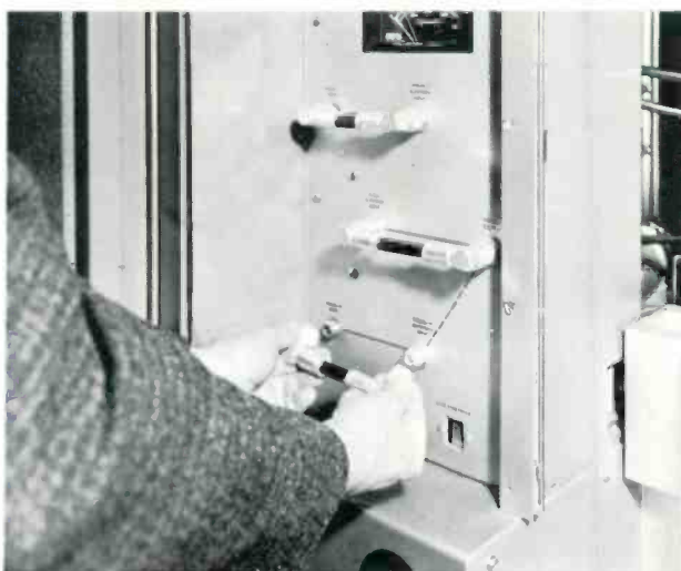
Unique patch panel permits instant use of visual PA for aural PA.
