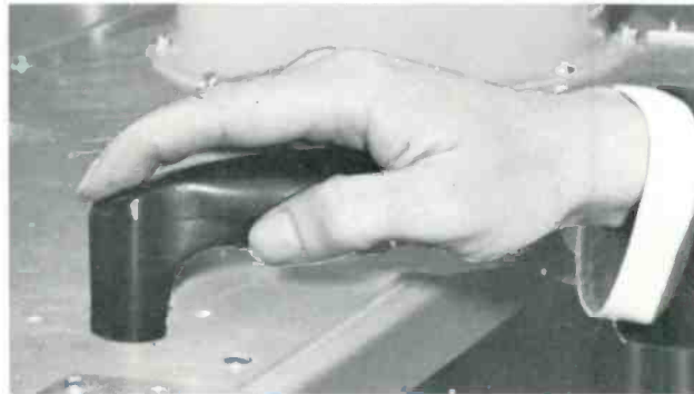
Switch for each klystron cabinet disconnects cubicle from operating transmitter.
