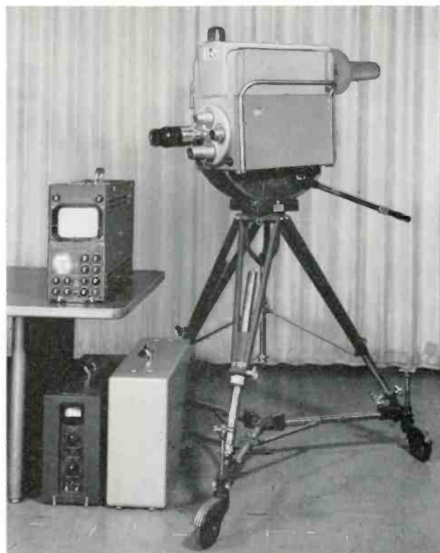
TK-14 Field Camera Chain showing Field Camera Control on table, TY-31A Field Power Supply and Field Case containing Focus Current Regulator and Electro-magnetic Orbiter Generator beside camera and viewfinder mounted on field tripod and dolly.
