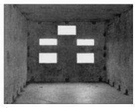
Connection plates are cast into the concrete panels. All panel connections are welded together.
