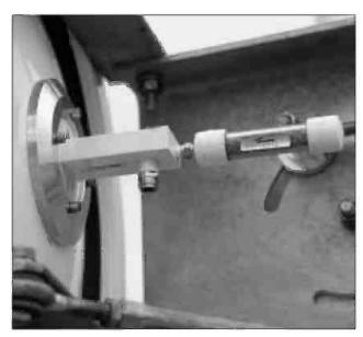
Static Desiccator SD-001 attached to Microwave Antenna Feed.
