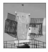
S- and C-Band Weather Radar Antenna/Pedestal
