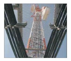
HELIAX elliptical waveguide is the optimum choice for most microwave antenna feeder systems. HELIAX is precision-formed from corrugated high-conductivity copper and has an elliptical cross section. The corrugated wall gives the waveguide excellent crush strength, light weight and good flexibility for ease of handling. A rugged black polyethylene jacket provides protection during handling and installation. A full range of waveguide sizes is available for application from 1.7 to 26.5 GHz.
