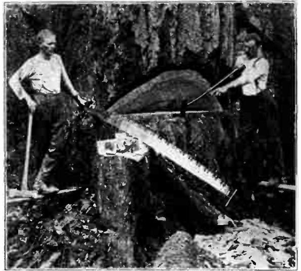
Showing how the Big Firs are Felled
