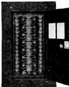
Standard Superba, with Doors over Fuses—Single Door Front
