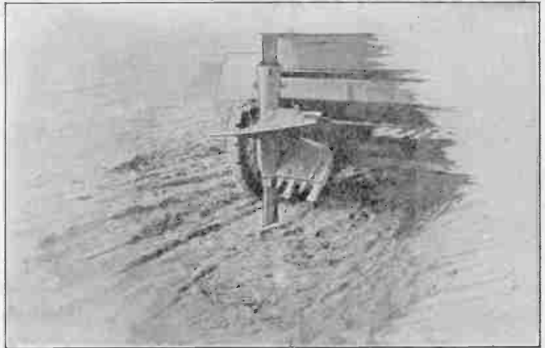
The Auger for Boring Through Shale
