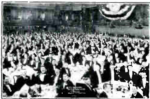
Public Address System in Use at Hotel Astor, New York
