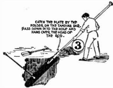
TO DRIVE THE ROD, DROP INSTALLING BAR IN THE HOLE AND DRIVE THE ROD WHILE HOLDING IT IN THE SAME PLANE AS THE BAR. NOTE-ALWAYS USE A NEVER CREEP MAUL. THE WOODEN FACE PREVENTS INJURY TO GALVANIZING.
