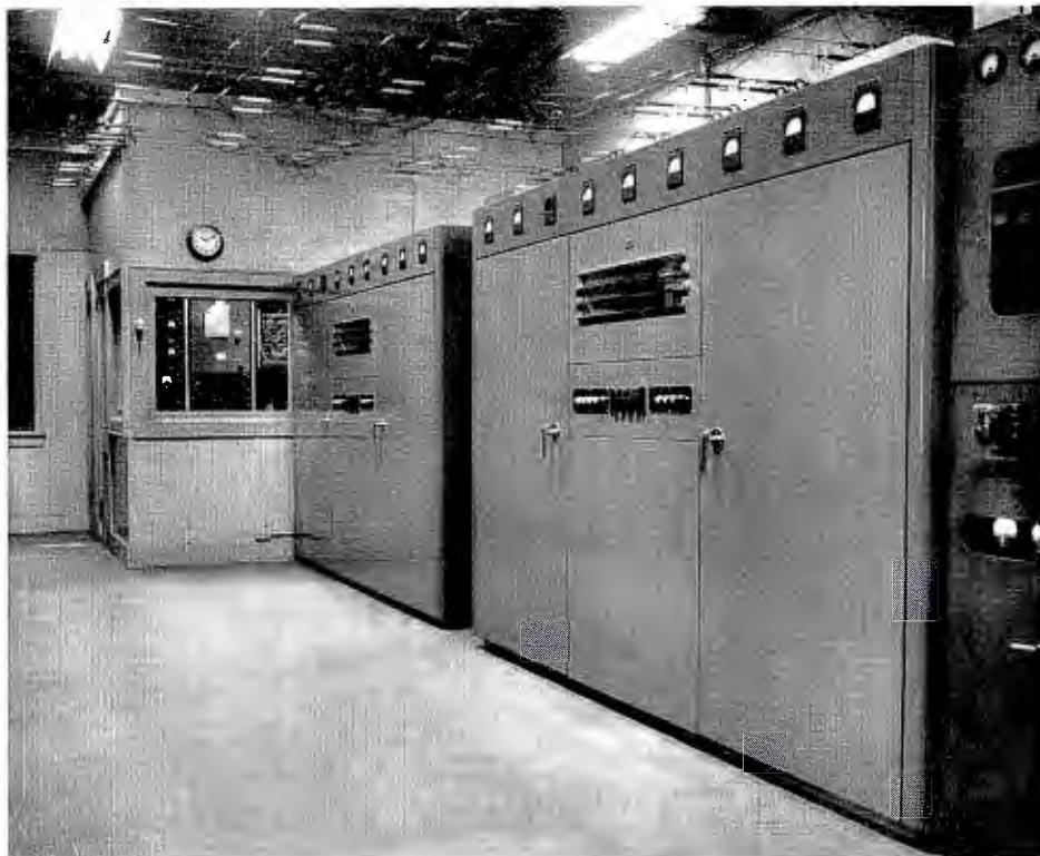
Below, duplicate HF-10TX 10,000 watt telegraph transmitters installed at Press Wireless, Inc., Hicksville, L. I., New York.
