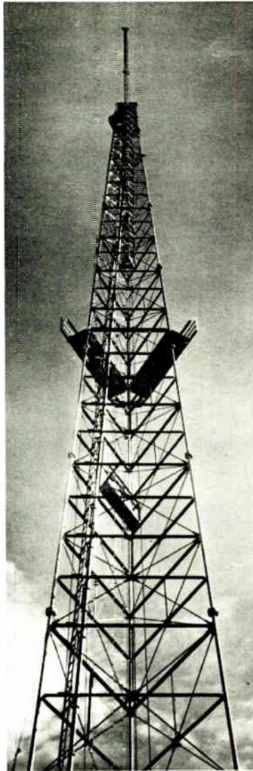
At Rochester, N. Y., this self-supporting tower gives the WOKR antenna 306.5' elevation above the ground.
