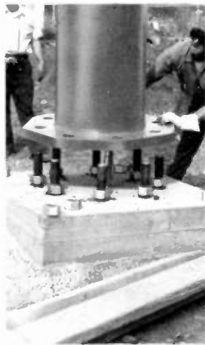
Pole in position to be lowered on plumbing nuts.
