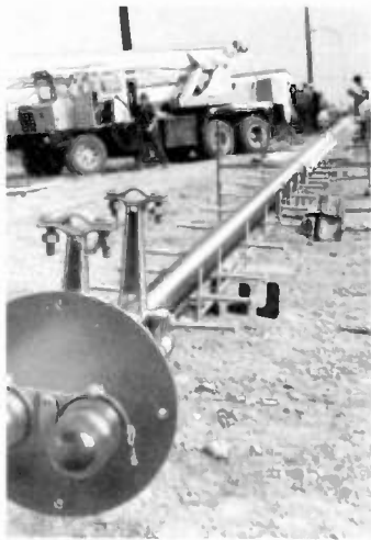
Pole and accessories assembled on ground prior to erection.
