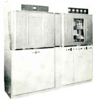
ABOVE, 1 kw phasor with rear doors open. AT RIGHT, 1 kw two-tower phasor installed with Collins 20V-2.
