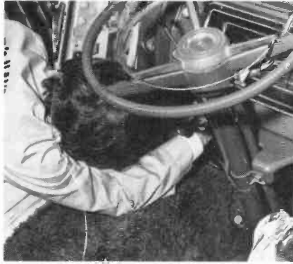
Using a #29 tap drill bit, drill a small hole under the carpet and through the fire wall. Through here you will run the power and grounding wires.
