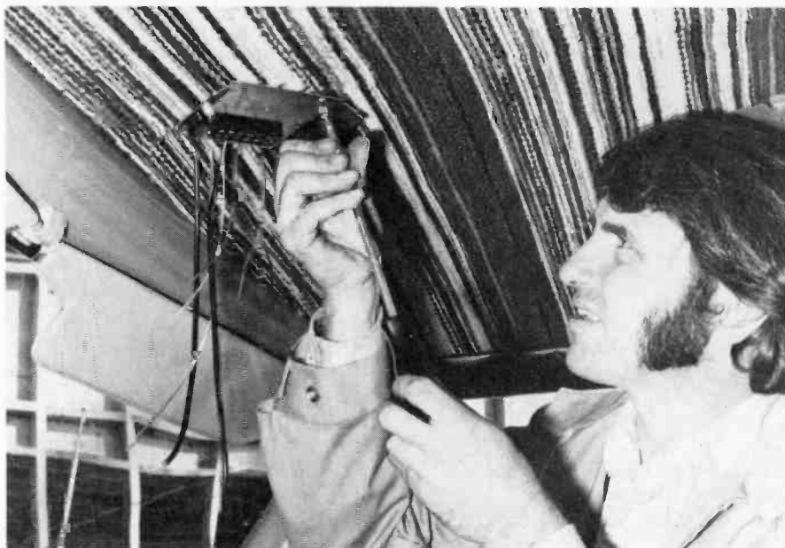
Make sure you know what you're drilling into. A high-speed drill can easily tear up other electrical wiring or even worse, bore through the van's roof!
