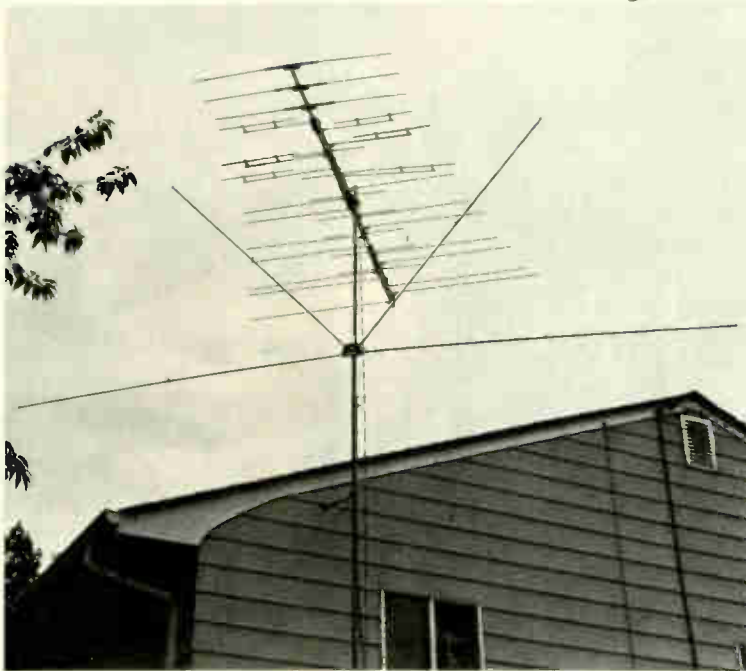
Omega CB antenna installed below TV antenna
