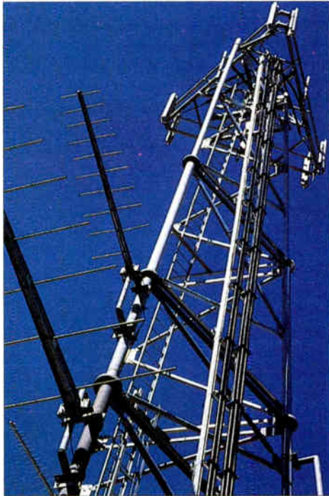
Figure 4. Lost elements on an antenna can degrade its performance, not only in gain, but in frequency response as well. Note the missing element on the top antenna.
