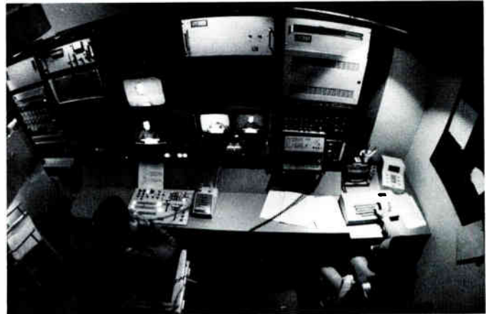
UA-Columbia's channel 3 control room.
