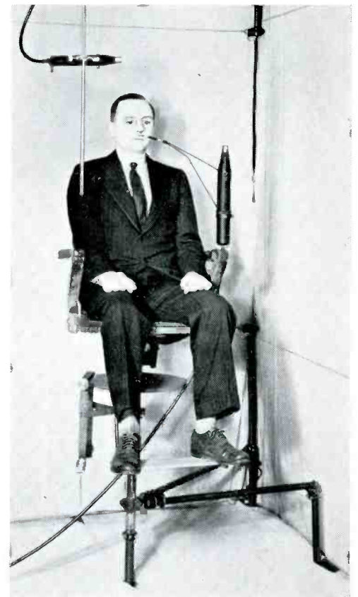
Fig. 1—Arrangement of speaker and microphone for distribution measurements
