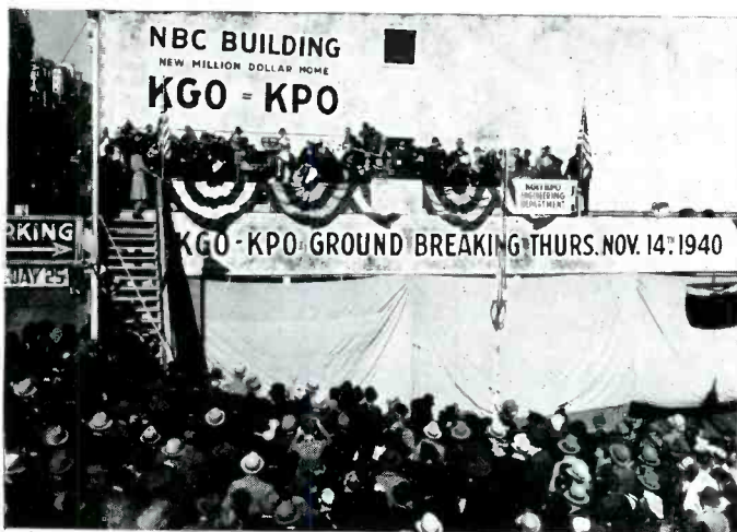
Every member of the KGO-KPO staff, including artists and musicians, joined their general manager, Al Nelson, in breaking ground for the new NBC Building while thousands of spectators covered the property and blocked two adjoining streets.
