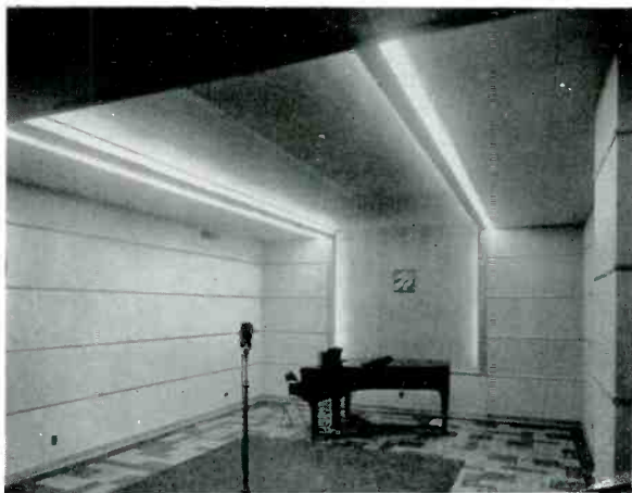
By moving talent practice rooms to the next floor above, WLS made room for the addition of this new studio D, with latest acoustically treated walls and ceiling, tile block floor and concealed, fluorescent lighting.
