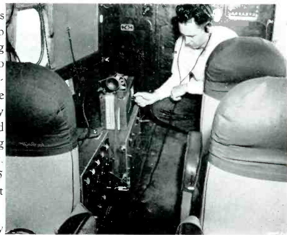
Installation of the ND-20 transmitter. One seat was removed and the equipment tied down with webb straps. Transmission line from the antenna fed in through fresh air intake. Converter and storage batteries not shown here were in baggage compartment, in the nose of the ship. Vern Andrews operating
