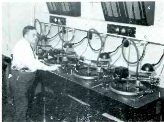
Hollywood Recording Room—Mort Smith, in charge of Hollywood Recording, looking over a "Take." Note manometer for measuring vacuum behind Mort, also vacuum control ring at right end of vacuum equipment housing. These feed mechanisms being replaced by Presto 8A as this goes to press.
