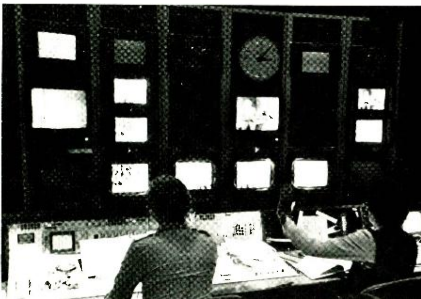
This newly refurbished control room with its state-of-the-art Grass Valley switcher can be used with various studios in the 10-acre KTLA studio complex in Hollywood. The 100,000 square-foot, 9-studio lot has been designed so that control rooms and cameras can be readily patched to different studio and control-room locations. (Photo by Ron Whittaker)
