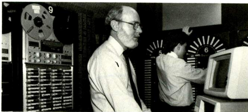
WQXI's chief engineer Tom Giglio (in foreground) accesses the station's IGM-SC automation controller via a PC, while program director Fleetwood Gruver III looks over one of the facility's IGM GoCarts.
