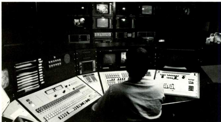
The Grass Valley Group 1600-4S/M-200 master control/automation system makes life easier for operators at KPTV, in Portland, OR.
