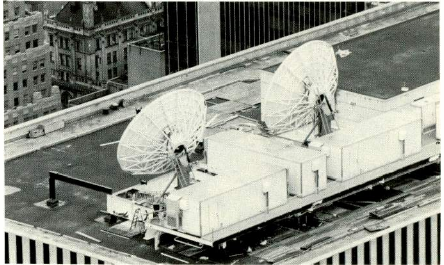
NBC's Skypath/New York master earth station, atop a Manhattan skyscraper. Each antenna transmits four video channels, in Ku-band.
