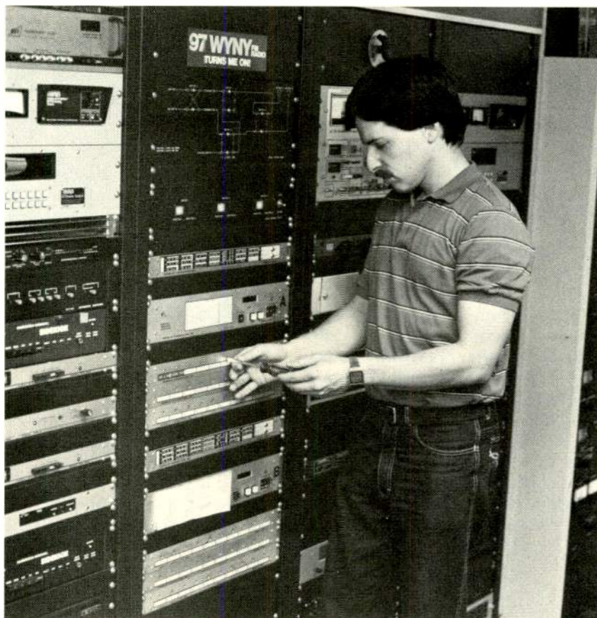
Engineer Lloyd Prezant of New York FM station WYNY stands to the right of an eye-level Harris RF status panel. The panel gives at-a-glance diagnosis of the status of the RF flow of the station's two Harris 25K transmitters.
