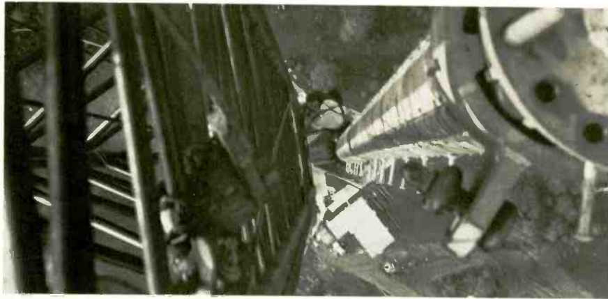
KLRN-TV's antenna and tower at New Braunfels, TX.
