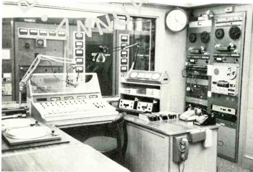
WANN-AM in Annapolis has just installed a Radio Systems ESA-10 console and Revox PR-99 ATRs as part of its ongoing conversion to stereo.
