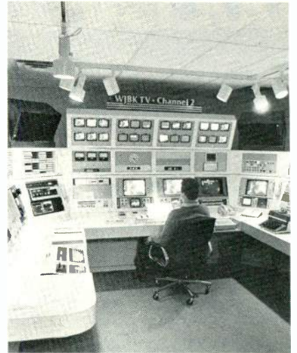
In WJBK's master control, a custom console houses the GVG 1600-4S MC switcher that automates on-air operations.
