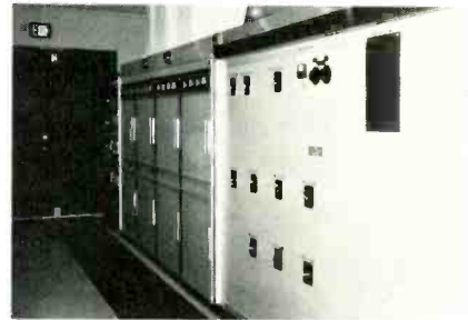
A Delta C-Quam ASE-1 exciter and ASH-1 modulation monitors have been added to the 50 kW McMartin BA-50K transmitter at left. In the foreground is the four-tower phaser from Vector Technology.
