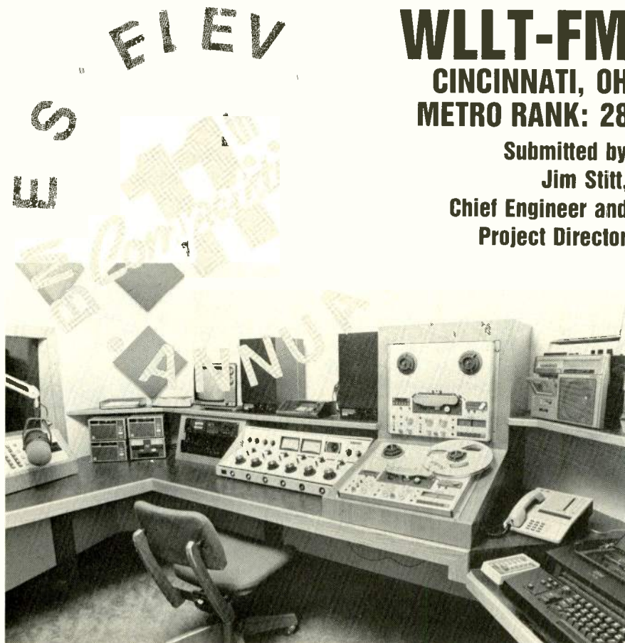
The WLLT newsroom is equipped with an Autogram console, three ITC-99B carts, two Studer-Revov PR-99B tapes, Technics cassette, Yamaha tuner, and Fostex speakers.
