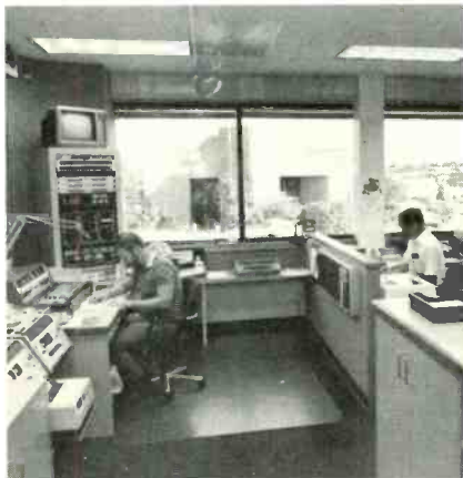
The stations' newsroom features a main anchor position (left) that uses a Howe Audio Model 7500 console, two Otari MTR-10 two-track machines, and three ITC Delta III three stack cart decks with record amplifiers.
