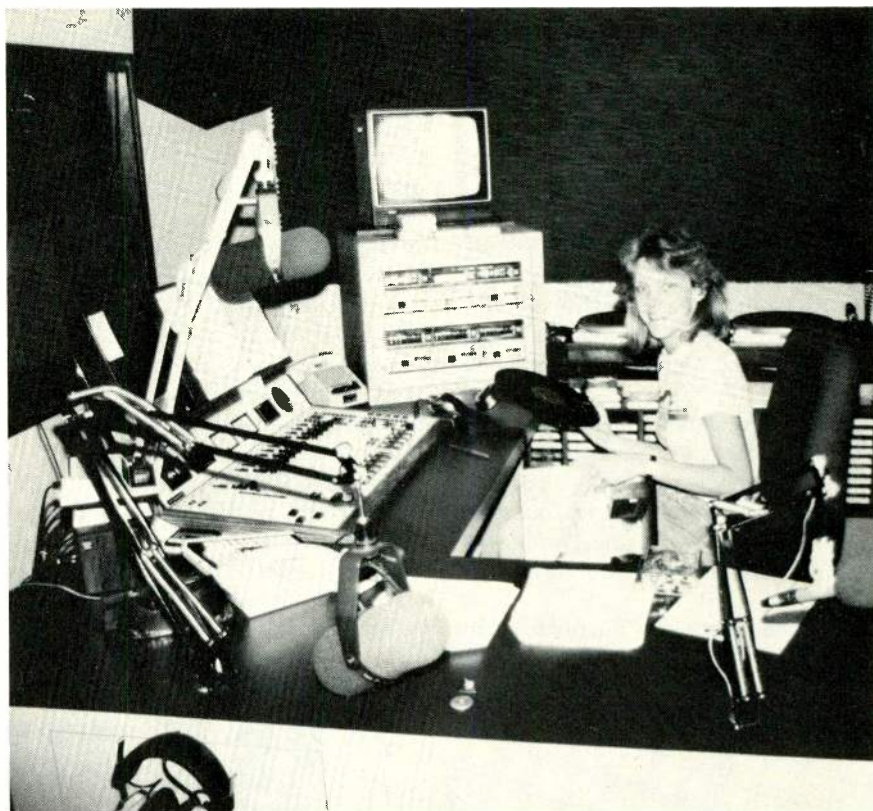
DJ Sharon LePere in KSJL's air studio, which features a BMX II 14 fader board, six Tomcat play-only cart machines, and two Technics turntables.
