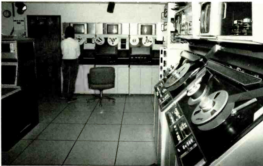
WRGT's equipment room has two RCA-600 two-inch machines, three RCA TR-800 one-inch decks, 12 RCA HR-2As, and a host of Sony 3/4-inch decks.
