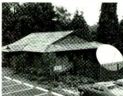
KTOL's 3.8-meter Comtech dish, right outside the station, provides insurance against closer satellite spacing in the future.
