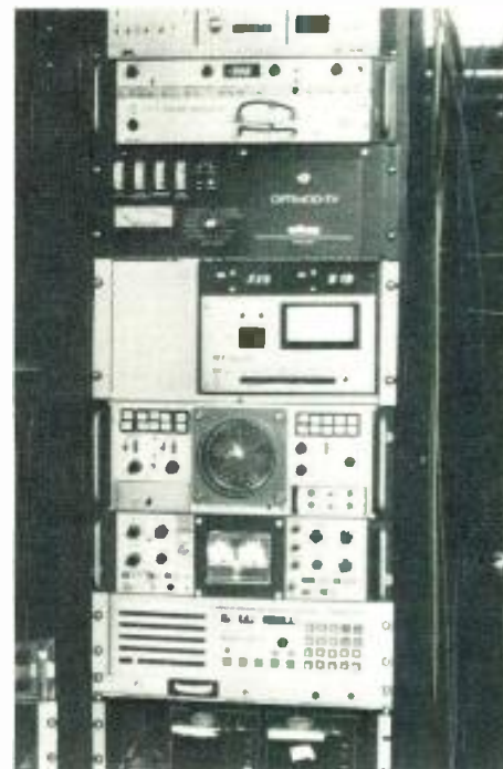
Master control hardware includes EBS receiver, demod, audio processor, frequency monitor, waveform monitor, vectorscope, and digital remote control.
