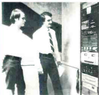
The AM control room monitor and control devices include an Orban Optimod AM, Harris AM 90 modulation monitor, Crown AM/FM house monitor amplifier, and remote metering and control
