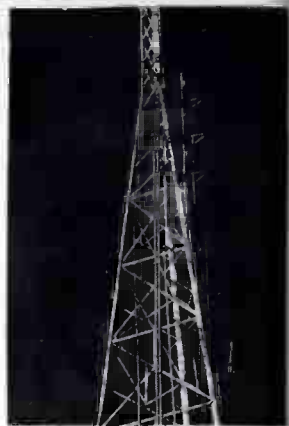
K101 antenna, used in air tests.
